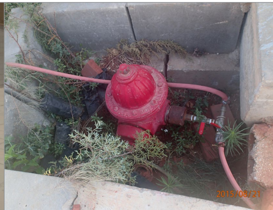
Figure 8B. Fire hydrant buried in concrete and tapped (Deficiency No. KAS-FP-150828-034) Source: DoD OIG, PO-TAD
