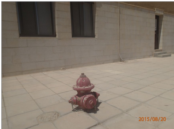
Figure 8B. Fire hydrant buried in concrete and tapped (Deficiency No. KAS-FP-150828-034) Source: DoD OIG, PO-TAD
